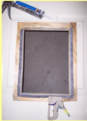
Use silicone caulking around trim kit for additional insulation. To quiet door closing staple 5/8" window felt to sides and bottom.
