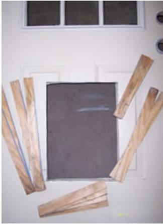
**If installing in a hollow core door**, use four strips of wood the same width as the hollow between the panels in your door. Position the wood so that they are flush with the edges of the hole. Either glue, nail or screw the strips. Frame the outside/inside hole with (2) inch by (1/4) inch lengths. Again, either glue, nail or screw to door surface as the photos illustrate.
