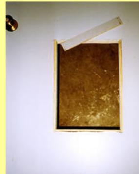
Steel door: Note hole is cut 3/4" (6/8") larger to allow for 3/8" thick wood inserts.
