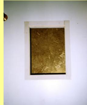
Frame the inside and outside of the hole on the door – use 3/8" cedar, pine or plywood strips — 1-3/4" or 2" wide.
